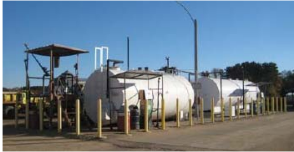
Figure 2. County Highway Garage Diesel Tanks
