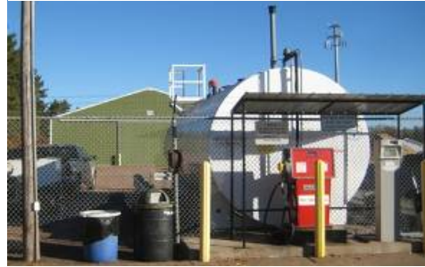
Figure 3. County Unleaded Tank
